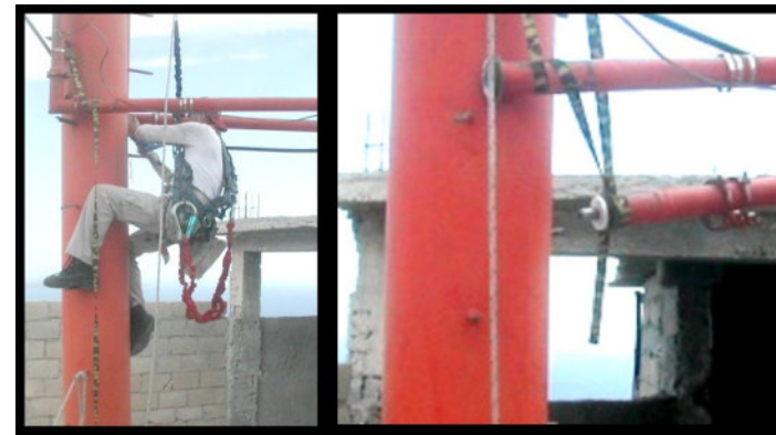
Joe Francis working on the feed lines.
