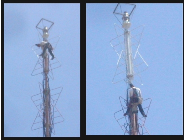
Joe Francis working on the beacon.
