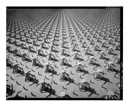
**This was in last months Ham Hum.** A close up picture of the hundreds of crossed-dipole elements on the sides of the early warning system developed in 1980 to detect and characterize a sea-launched ballistic missile attack against the United States.
