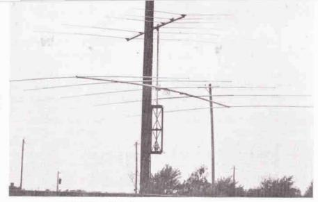
20-30 MHz KLM Log Periodic, and the new 5 el. Telrex 20 meter beam.
